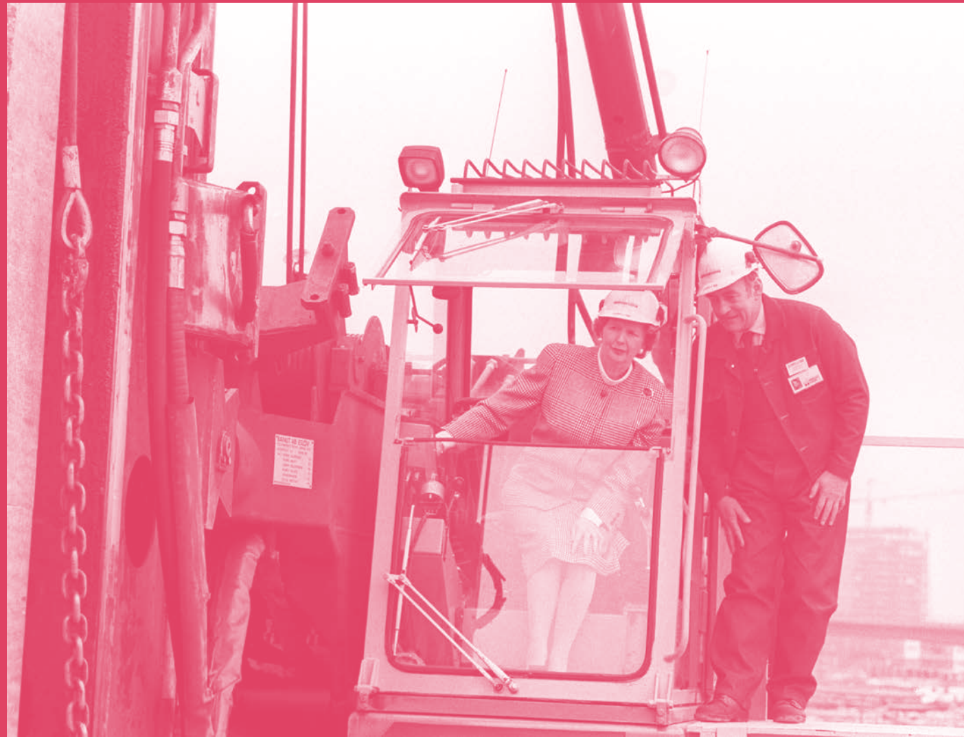
Prime Minister Margaret Thatcher, under tuition of a pile-driver operator, helping construction work on the Founders Court development at Canary Wharf © PA Images / Alamy Stock Photo
